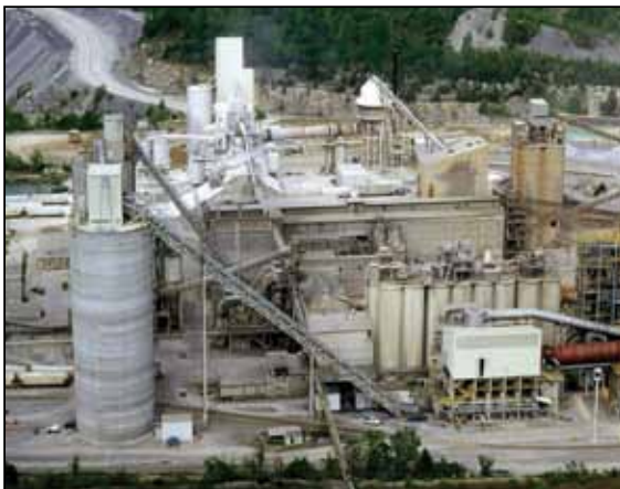
Safety first at this high efficiency cement plant.
